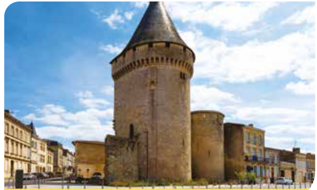
Grand Port Tower, Libourne ©Getty Images/JackF
